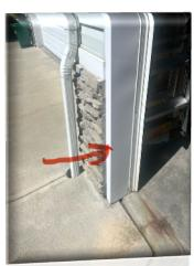
We are also looking at fixing or replacing the cladding around garage doors. Capping is a cladding or wrapping of aluminum sheeting over exterior wood trim. Your existing wooden garage doorframe is custom-fitted with aluminum sheets that are custom-cut and formed. We have seen quite a few frames that are rusty and in need of attention.
